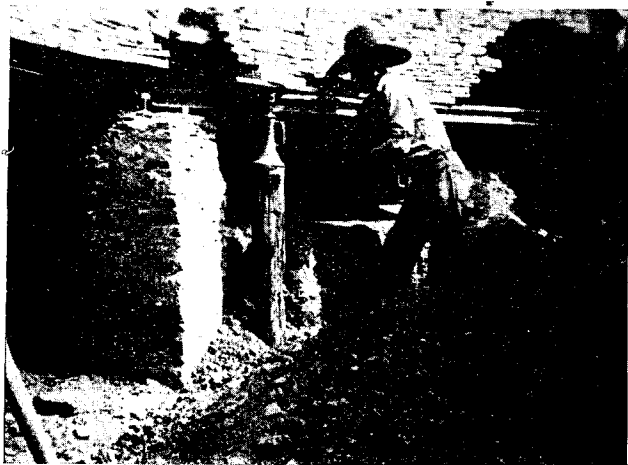
Plate II—Support Work of "East Tower" Section in Progress
