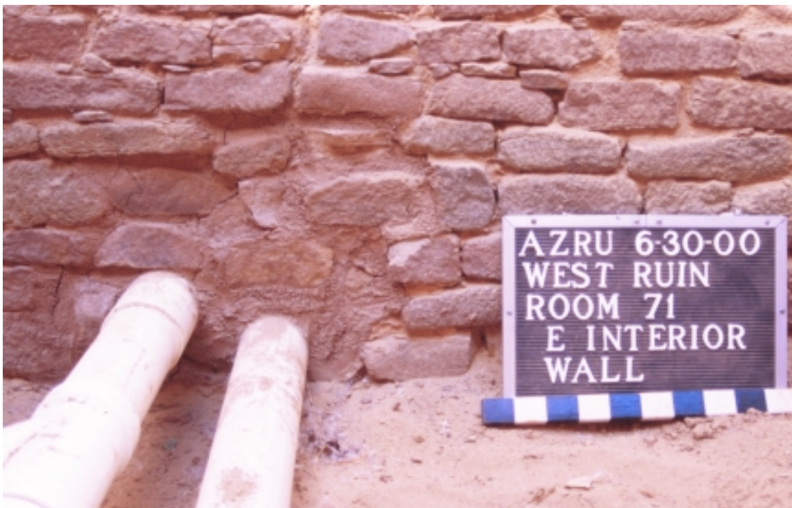
Figure 01J. East interior wall, looking northeast, after masonry closure around Perforation 2000-01.
