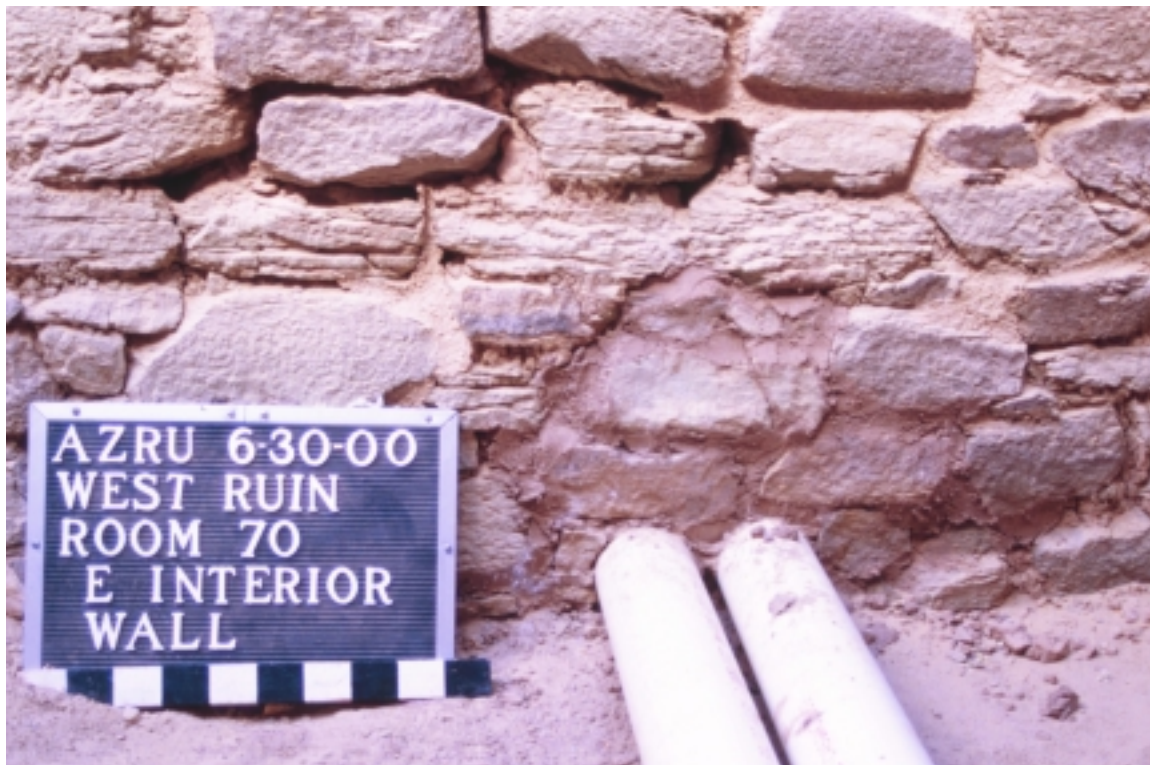
Figure 05G. East interior wall, looking northeast, after masonry closure around Perforation 2000-05.
