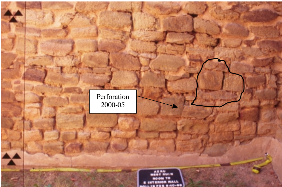
Figure 05D. East interior wall of Room 70, looking northeast at location of wall perforation that was opened during FY-00 backfilling project. Pre-backfill photo taken June 10, 1999.
