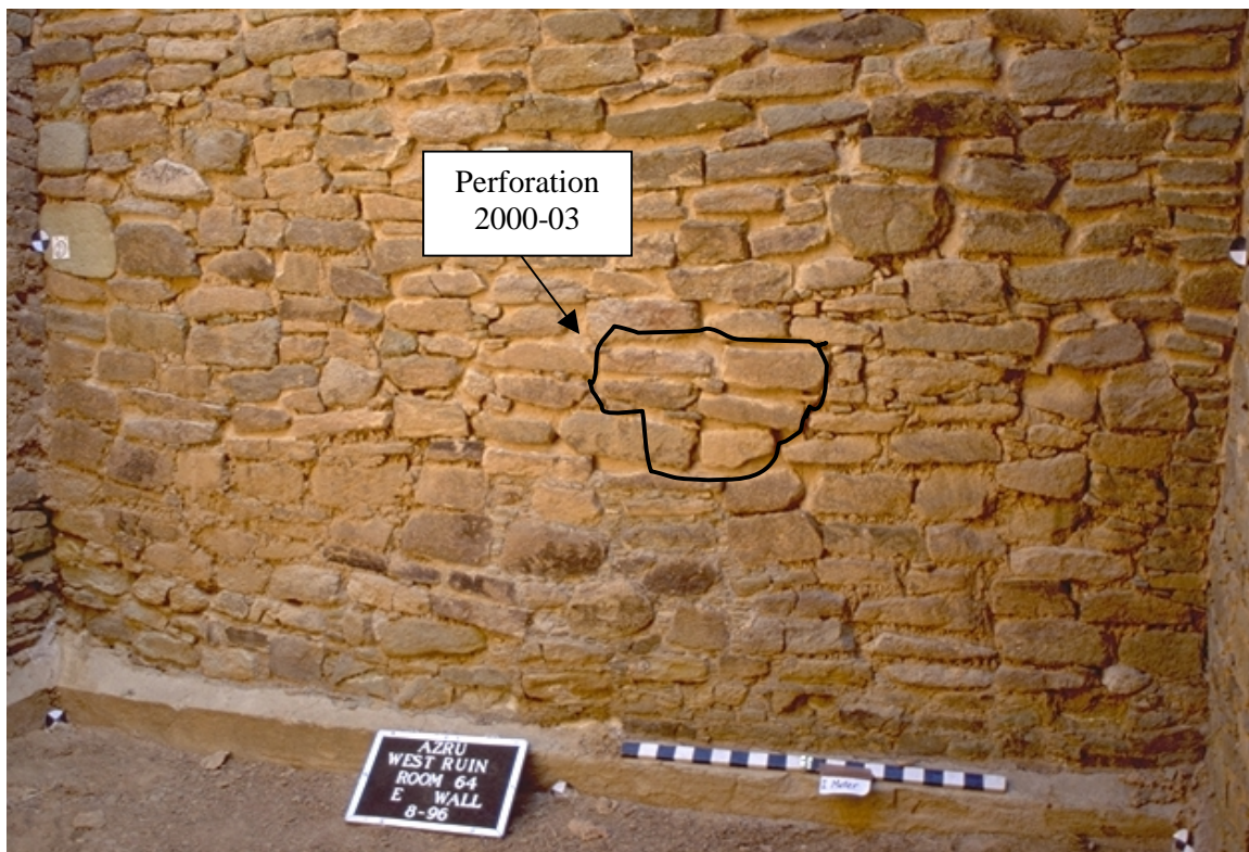
Figure 03D. East interior wall of Room 64, looking northeast at location of wall perforation that was removed during FY-00 backfilling project. Pre-backfill photo taken August 1996.
