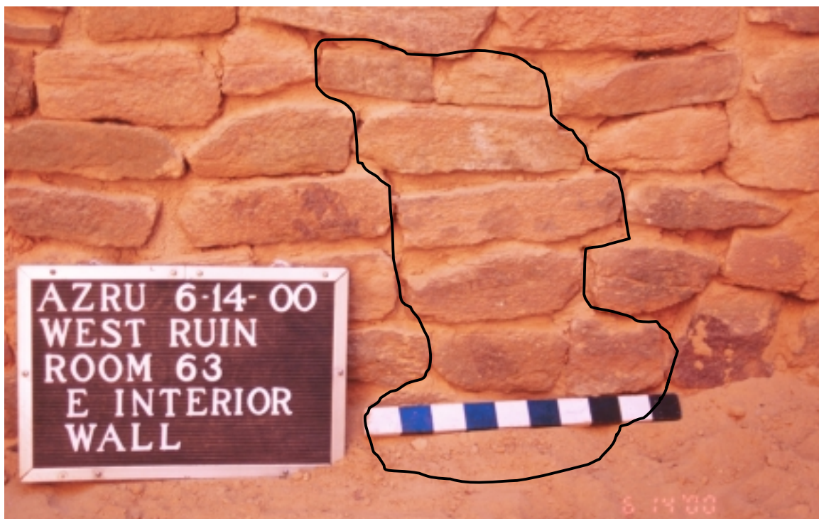
Figure 2F. East interior wall of Room 63, looking northeast, prior to removal of Perforation 2000-02 on June 14, 2000. Perforation is outlined.
