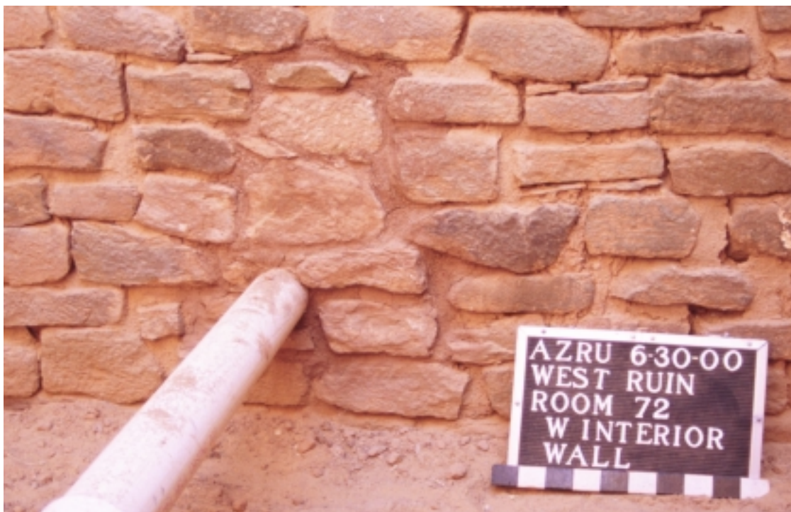
Figure 02D. West interior wall, looking southwest, after masonry closure around Perforation 2000-02.
