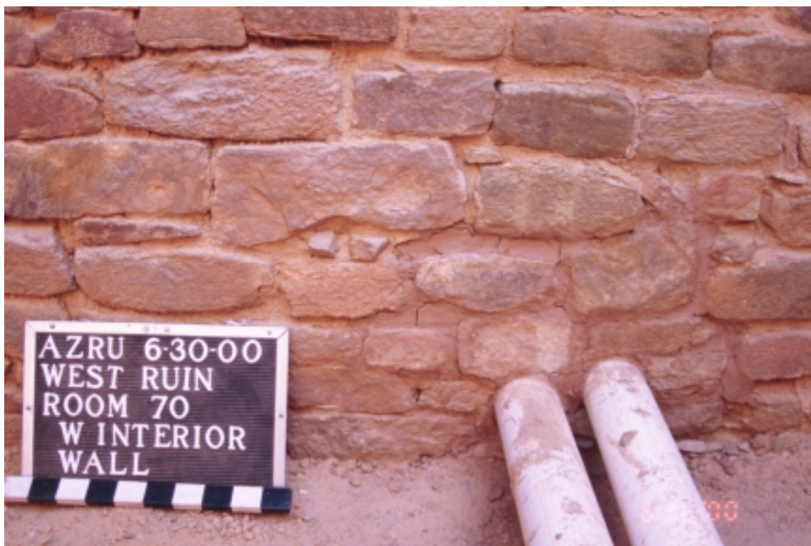
Figure 01D. West interior wall, looking southwest, after masonry closure around Perforation 2000-01.
