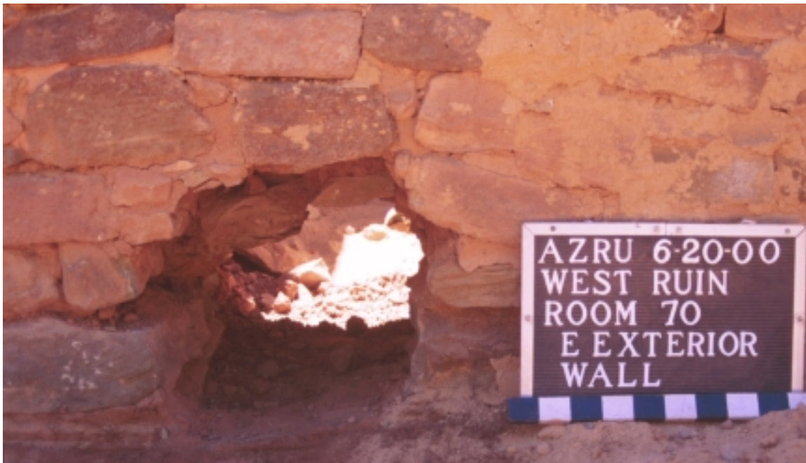
Figure 05C. East exterior wall of Room 70, looking southwest, after initial wall penetration.
