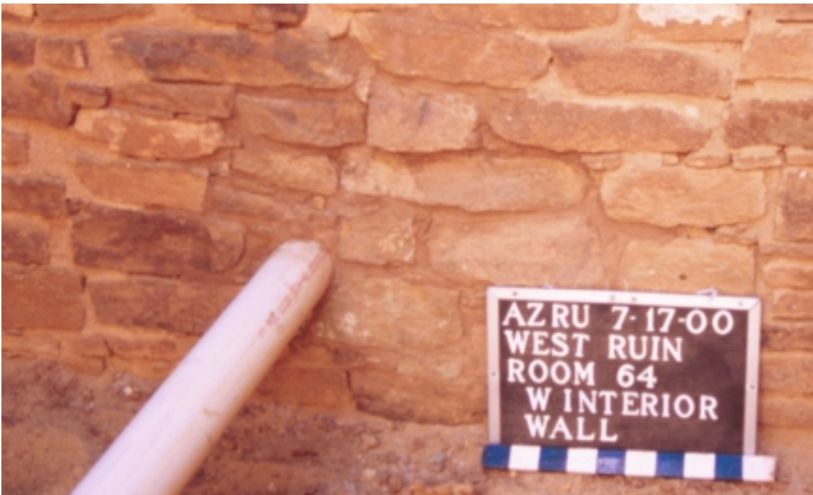
Figure 04D. West interior wall, looking southwest, after masonry closure around Perforation 2000-04.
