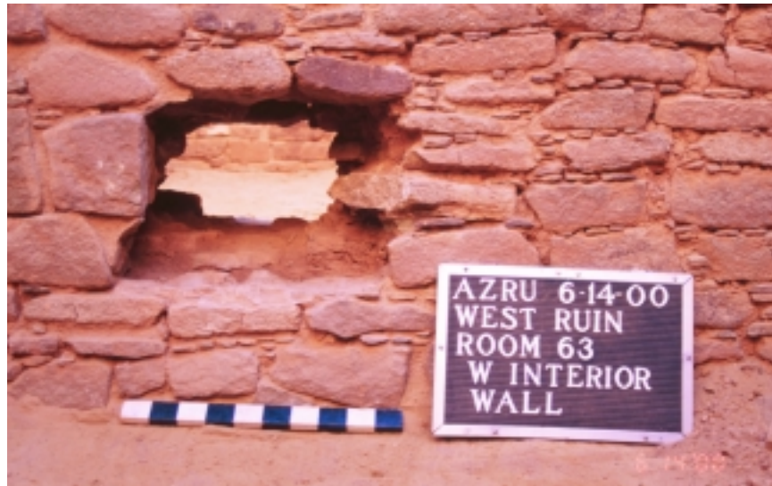
Figure 03C. West interior wall of Room 63, looking southwest after initial wall penetration on June 14, 2000.
