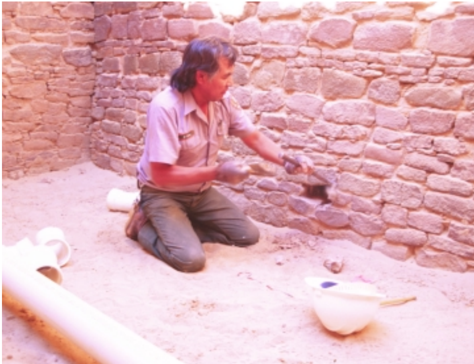
Figure 01G. James Brown chiseling out building stones for Perforation 2000-01 on east interior wall of Room 71.
