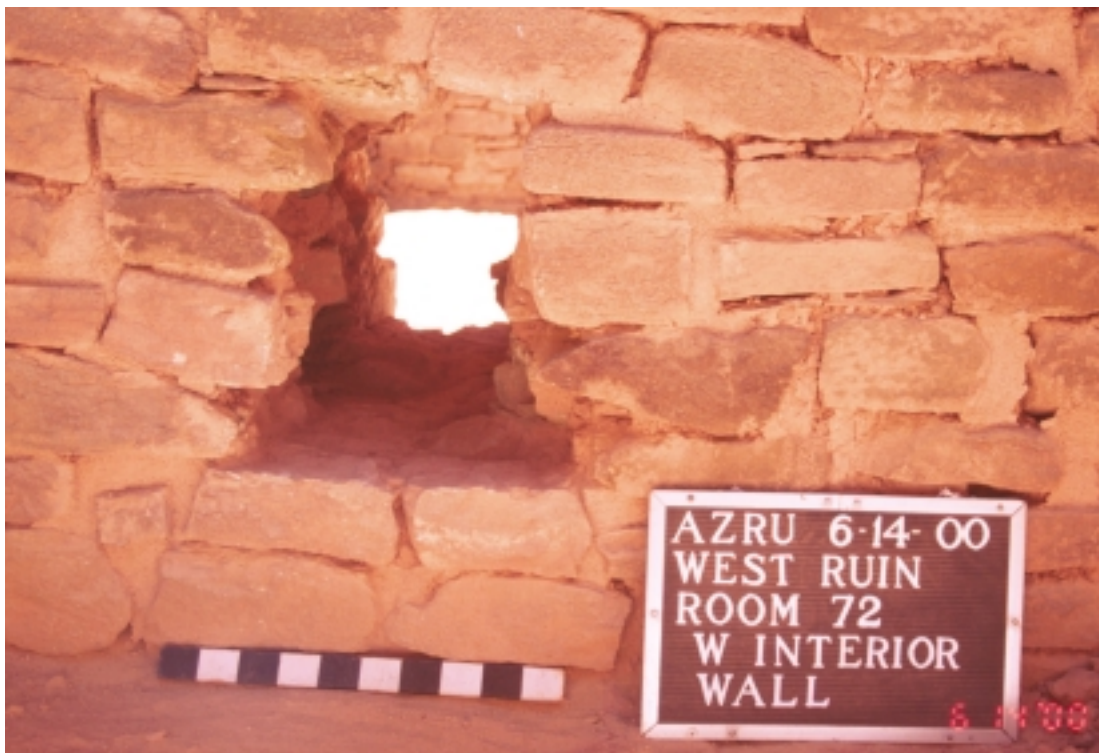
Figure 02C. West interior wall of Room 72, looking southwest, after initial wall penetration on June 14, 2000.
