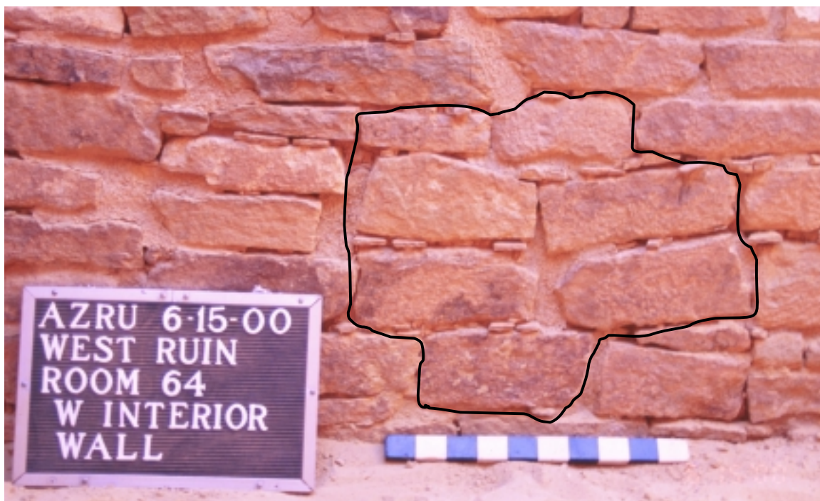
Figure 04A. West interior wall of Room 64, looking southwest, prior to removal of Perforation 2000-04 on June 15, 2000. Perforation is outlined.
