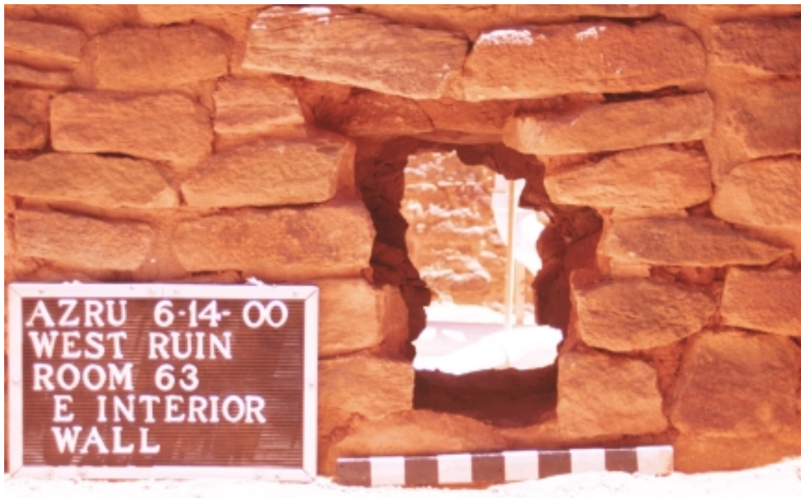
Figure 02G. East interior wall of Room 63, looking northeast into Room 72 through initial wall penetration on June 14, 2000.
