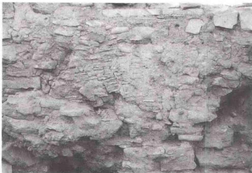
Figure 4.25. Room 7, close view of chinking in plugged Doorway 2 at the eastern end of the south wall (Chaco Project Neg. 19087)
