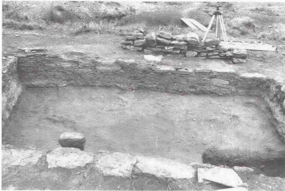
Plate 4.1. Room 1, Floor 1 and north wall. Note stone step in lower left of room and subfloor test pit in lower right (NPS 10484).
