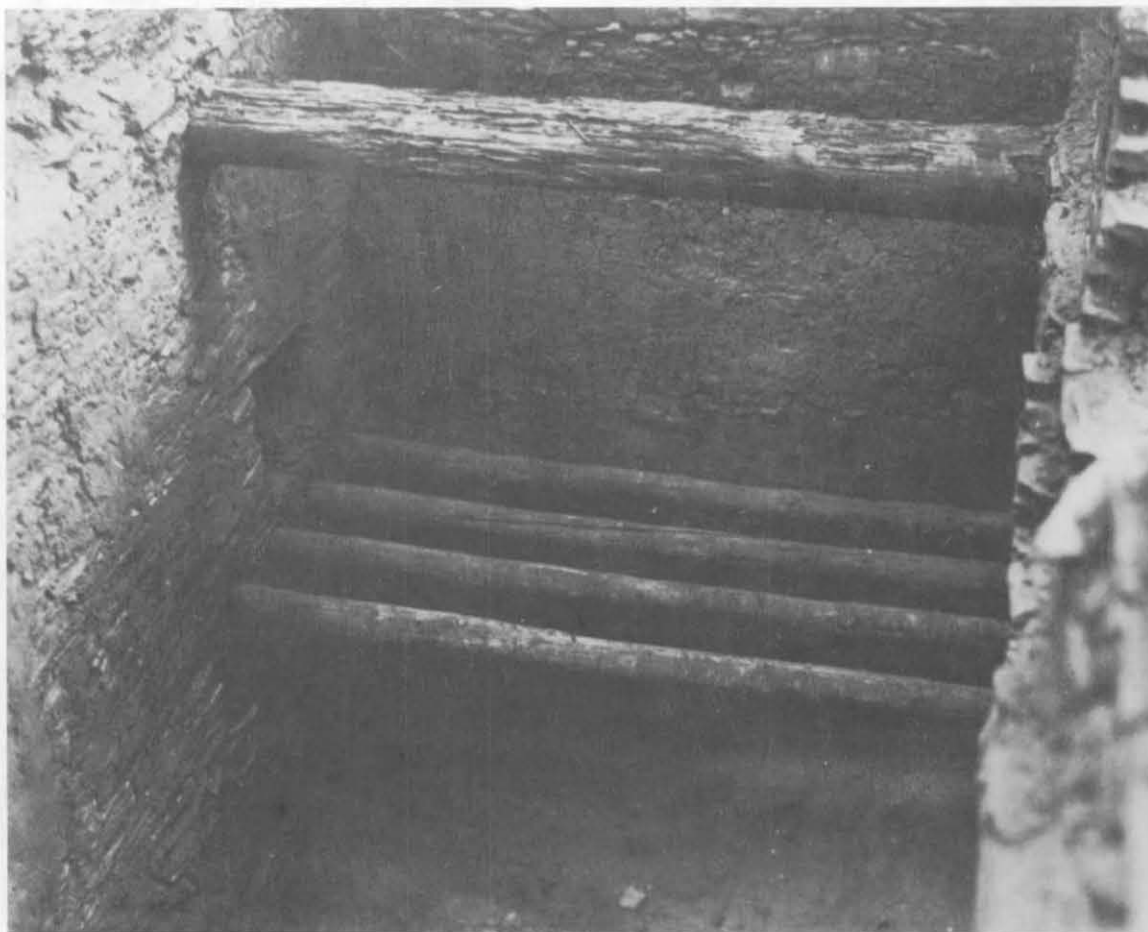
Figure 3.3. Primary beams of a room-wide platform, Room 48, Chetro Ketl (Reiter No. 1115.599, Chaco Center Archive No. 2176H).
