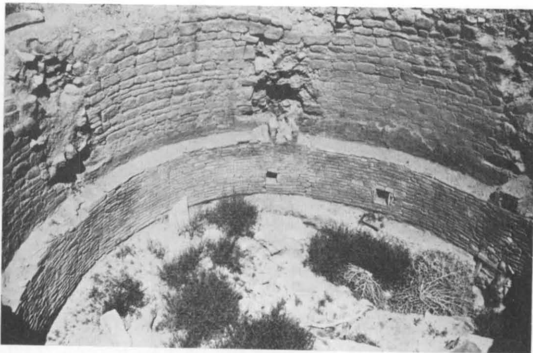
Figure 78. Ida Jean Chacoan structure. Fine slab and block masonry in Chaco-style kiva. Note horizontal log pilasters and sub-floor vent.
