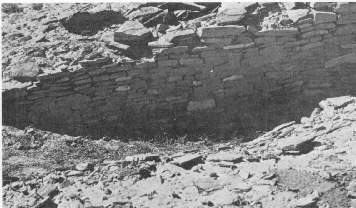
Figure 31. PS-3, small house. Exposed core and veneer masonry in west wall of pothunted room.
