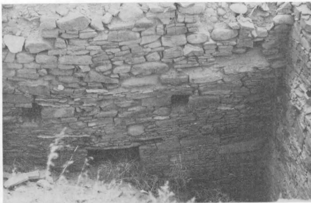
Figure 67. Site 41. Partially excavated room in Chacoan structure. Square holes above doorway are primary beam sockets for first story roof/second story floor. Veneer stones are fire-reddened suggesting possible burning of structure.
