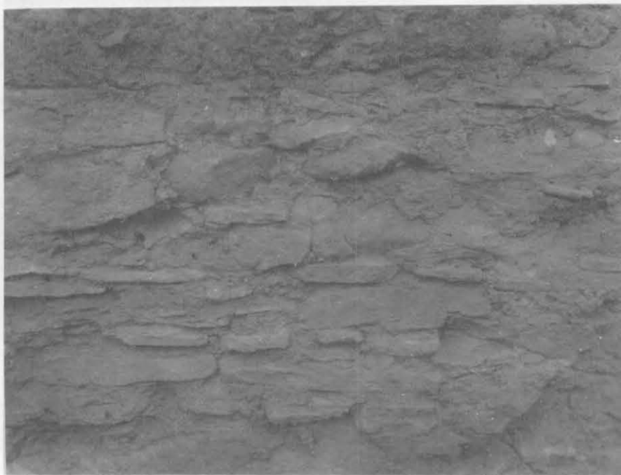
Figure 2.31. Interior of west wall, Room 11; detail of spall and unmodified tabular sandstone masonry
